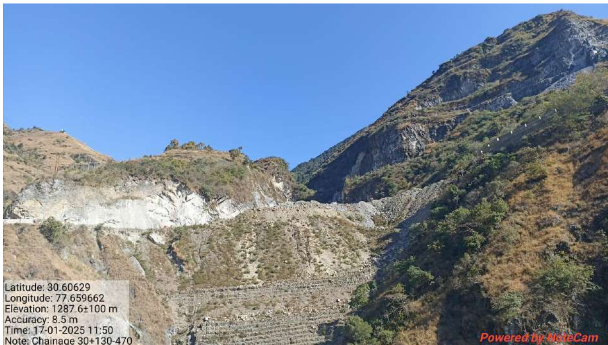
Refer photo at Page No. 4433 (Ch. 30+130 to 30+470): This is the designated dumping site and the dumping has been done with the concern/permission of the concerned department. Gabion wall was constructed at the toe to protect the dumping site.
