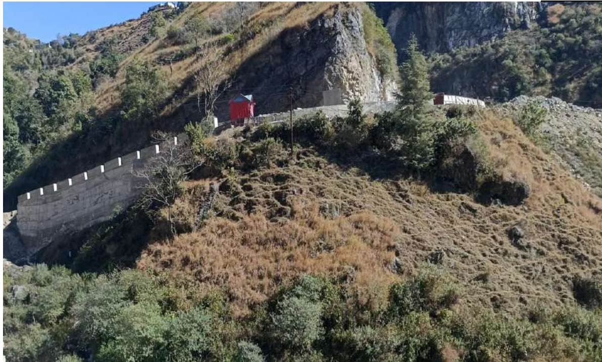
Refer photo at Page No. 4433 (Ch. 30+130 to 30+470): This is the designated dumping site and the dumping has been done with the concern/permission of the concerned department. Gabion wall was constructed at the toe to protect the dumping site.
